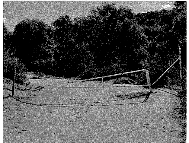
Access gate in need of repair.
