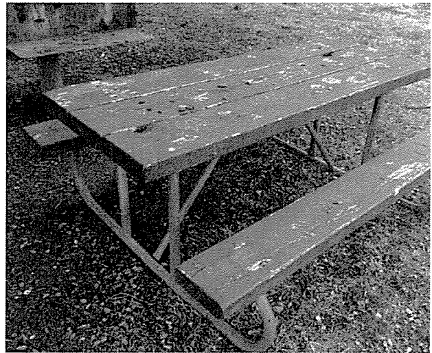
In need of sanding and a fresh coat of paint.
