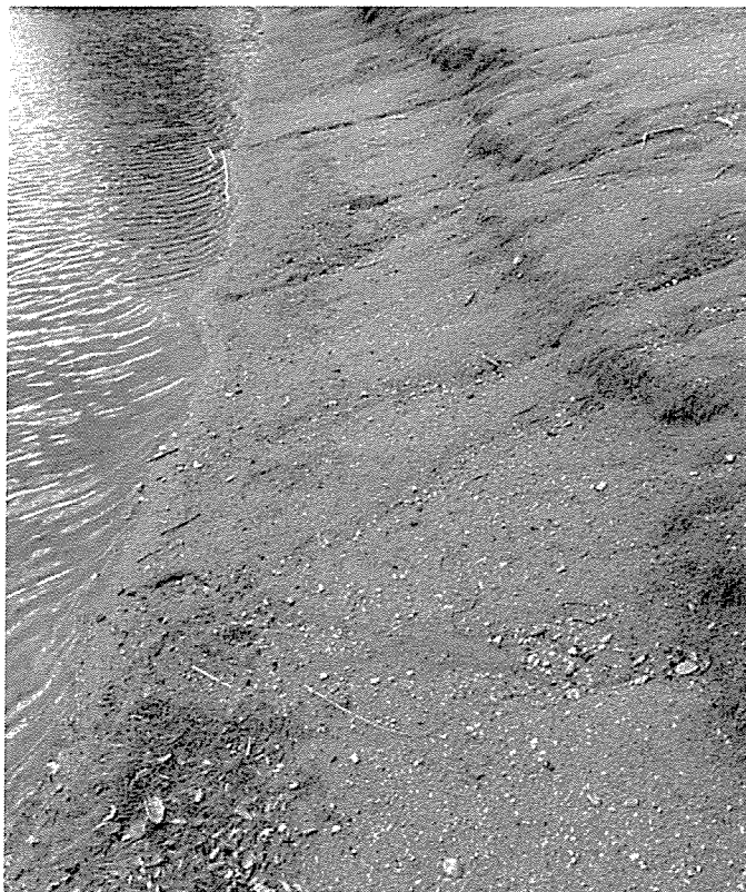
Erosion into the pond.
